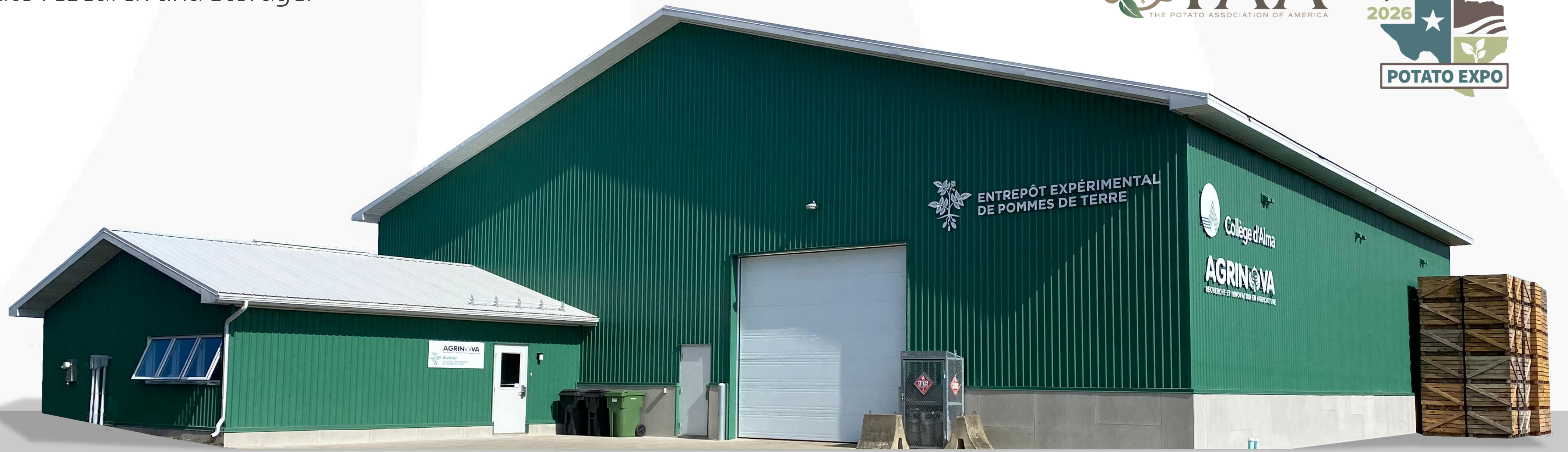
Our experimental potato storage facility in Québec (Canada).
